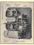
Fig. 33.-The mechanism of the Westinghouse Type RA demand watthour meter.
